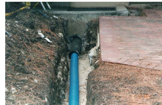
Double contained fuel piping
