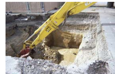
Excavating contaminated soils
